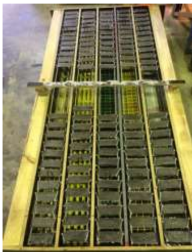
(a) Placement the reinforcement in the formwork,
