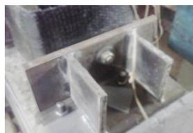
(b) Mechanical fasteners used to retrofit columns
