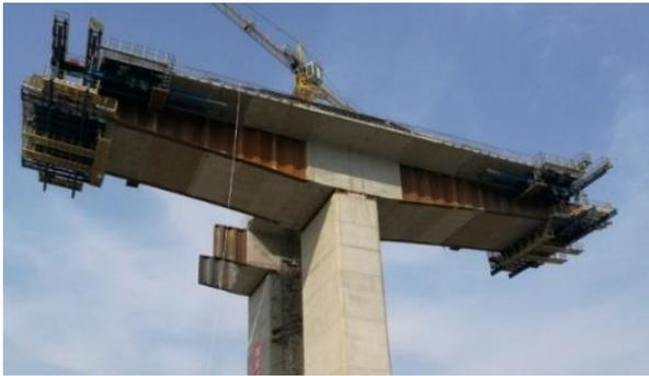
Fig. 4 Composite bridge on site (China) (Dong *et al.* 2017)
