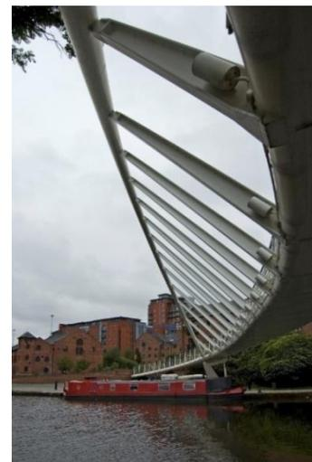
Fig. 27 Pinned end achieved by means of a tapered hanger with a very low-stiffness cross-section at an end. Merchants bridge, Manchester. Photo: Paul Harrop, geograph.org.uk
