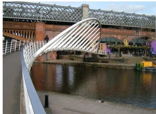
Fig. 6 Example of stiffened hangers. Merchants Bridge, Manchester. Photo: Clem Rutter, Wikimedia commons
