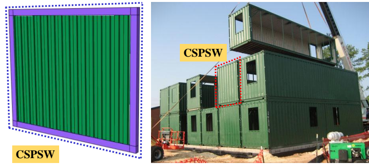
Fig. 1 C-SPSW in modular construction
