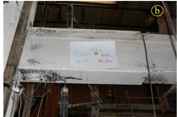
(b) Beam yielded at about 4% storey drift
