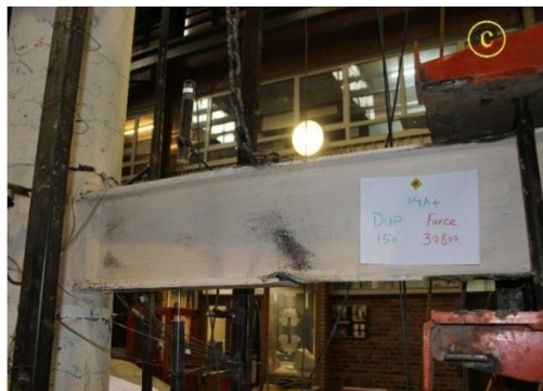
(c) Buckling of beam flange at about 5% storey drift
