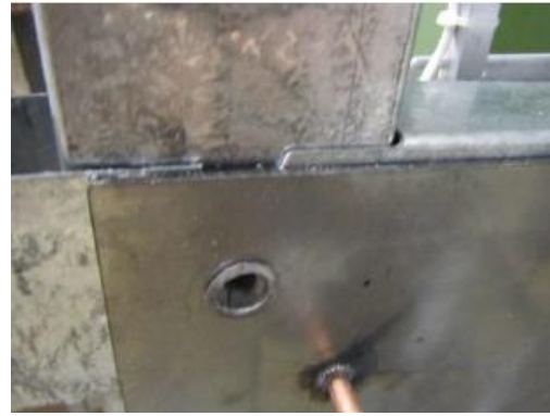
Fig. 25 Net section fracture of tension member in third moment connection test
