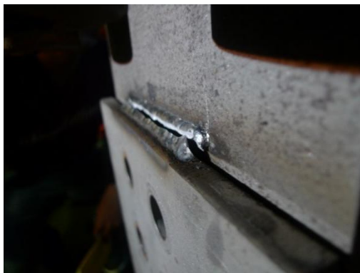
(a) Welded joint (crack angle = 45°)
