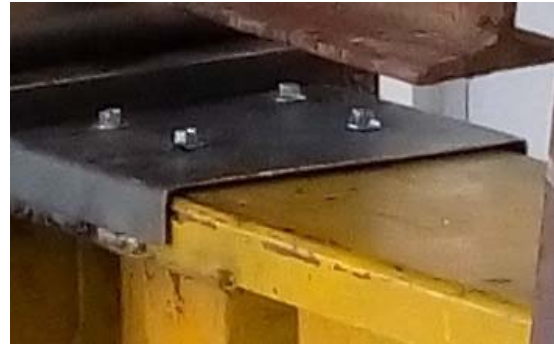
(b) Failure in Model A1
