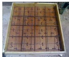
(b) RC formwork
