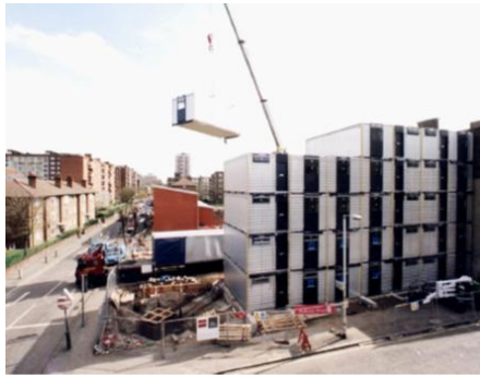
(a) Installation of a module building at London
