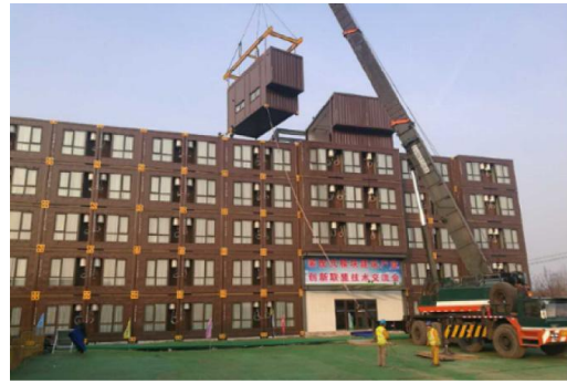
(b) A modular residence construction at Tianjin
