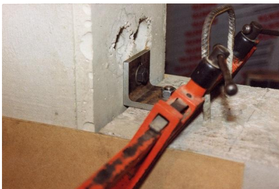
Fig. 10 Column connecting angle (connections ready for grouting)
