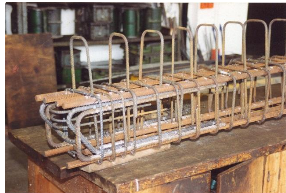
Fig. 8 Beam reinforcement for bolted billet connection
