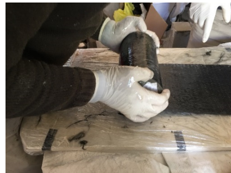
(c) Application and impregnation of the FRP fabric
