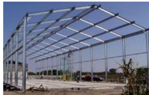
Fig. 1 Photograph of cold-formed steel portal frame after Wrzesien *et al.* (2015)
