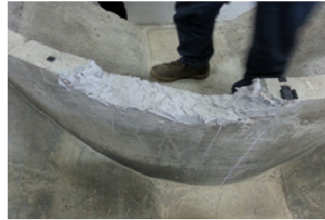
(b) Application of structural repair mortar using hand trowelling process
