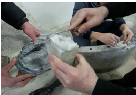
(b) Application of structural repair mortar using hand trowelling process
