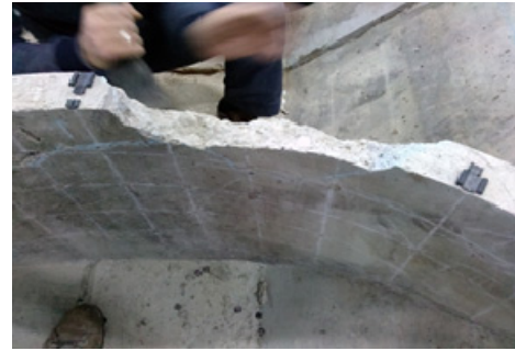
(a) Removal of the damaged concrete pieces
