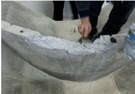
(b) Application of structural repair mortar using hand trowelling process
