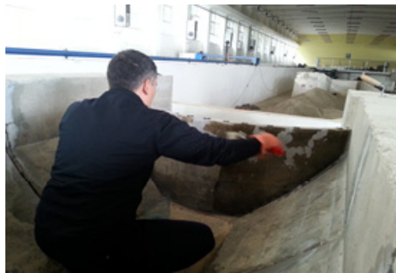
(a) Application of MBT-MBrace®Primer to the body surface
