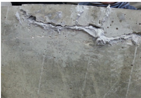
Fig. 12 Repair process of arch dam with epoxy mortar
