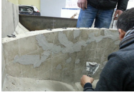
(e) Application of structural repair mortar on the surface of dam arc
