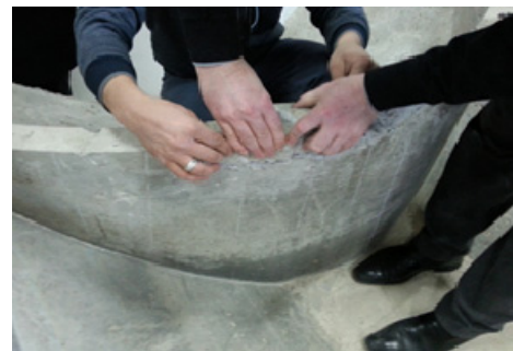
(b) Application of structural repair mortar using hand trowelling process
