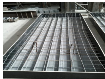
(b) Reinforcing and penetrating rebar fasten
