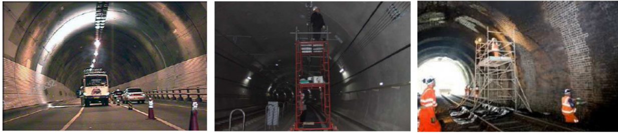
Fig. 2 Examples of tunnel temporary works
