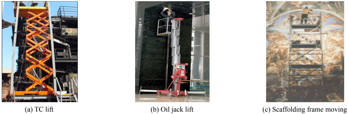
Fig. 3 Typical equipment of temporary works
