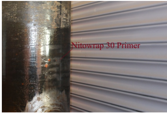
Fig. 4 Nitowrap 30 primer applied on the joint
