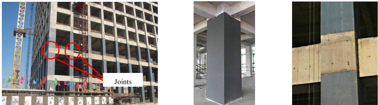
Fig. 2 Practical application of square TRC connection
