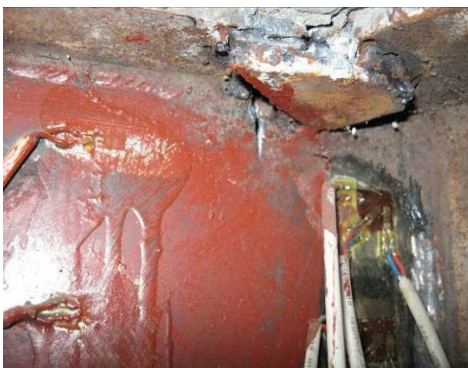
Fig. 6 Weld fracture at the box-girder flange
