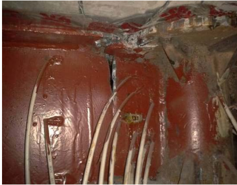
Fig. 8 Torn-crack in the web of box-girder
