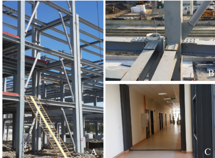
Fig. 3 Details of the separation, construction joint (A, B: View of the separation during the construction, C: view of the separation in the building in use)
