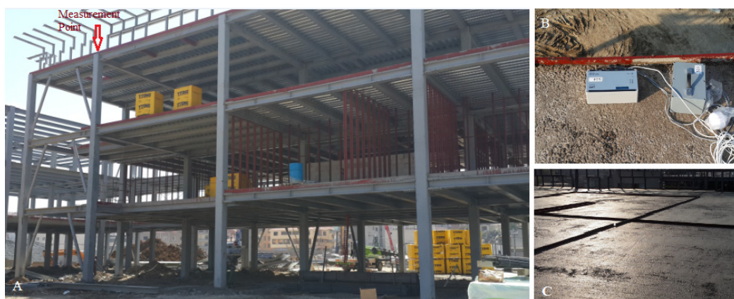
Fig. 8 The building on the third stage (A: general view, B: accelerometer in the measurement, C: completed concreting of the top floor)
