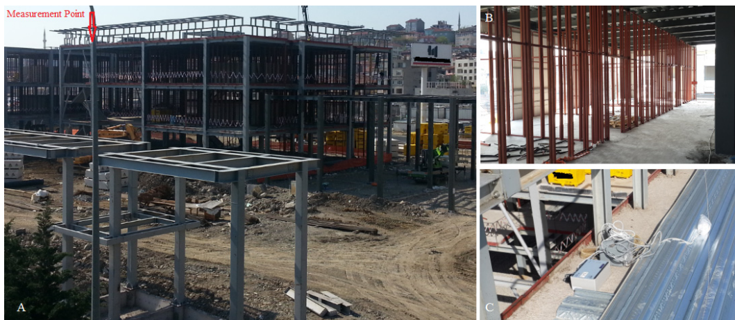
Fig. 10 The building on the fourth stage (A: composite slab after concrete pouring, B: accelerometer in the measurement, C: braces in Y and X directions on the ground floor)
