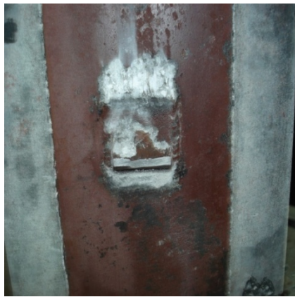
(a) Fractured channel in slab
