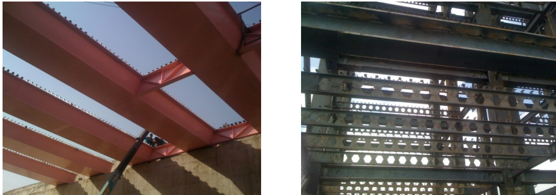
Fig. 4 Channel shear connectors in bridge and building structures
