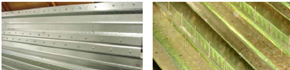
Fig. 3 Steel deck with screws drilled from the bottom side (left) and a view from the top side (right)
