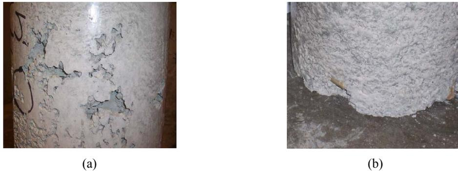
Fig. 1 Improper compaction of the cover concrete in Miller (2006)
