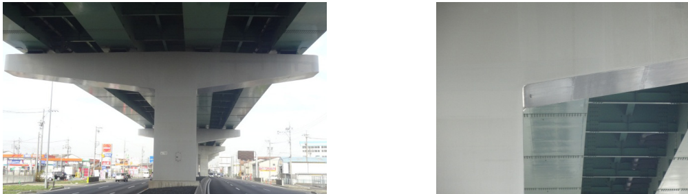
Fig. 3 Fillets with very small radius at beam-column connections
