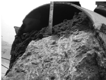
Fig. 1 A severe defect of inanity in the concrete filled steel tube of an arch bridge
