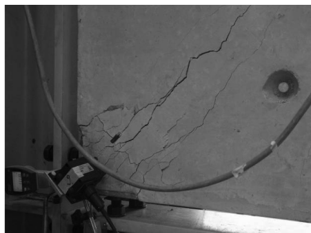
Fig. 10 Failure at panel corner with spalling and reinforcement yielding
