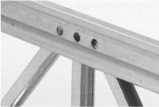
Fig. 1 Rosette-joint in a roof truss
