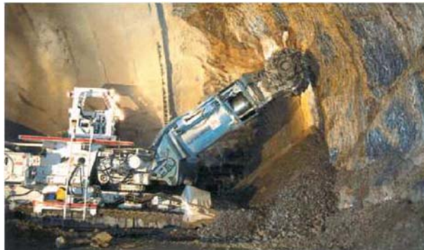
Fig. 20 Excavation with a roadheader
