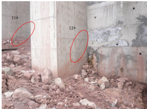
Fig. 6 Crack on the lower right side of No. 11 and No. 12 pile
