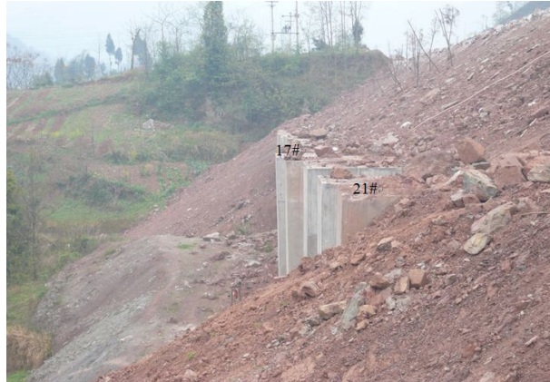
Fig. 5 The picture after anti-slide pile deformation
