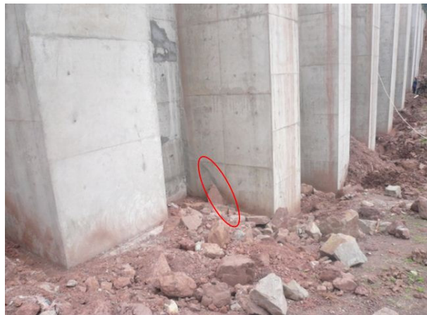
Fig. 7 Crack on the lower left side of No. 12 pile
