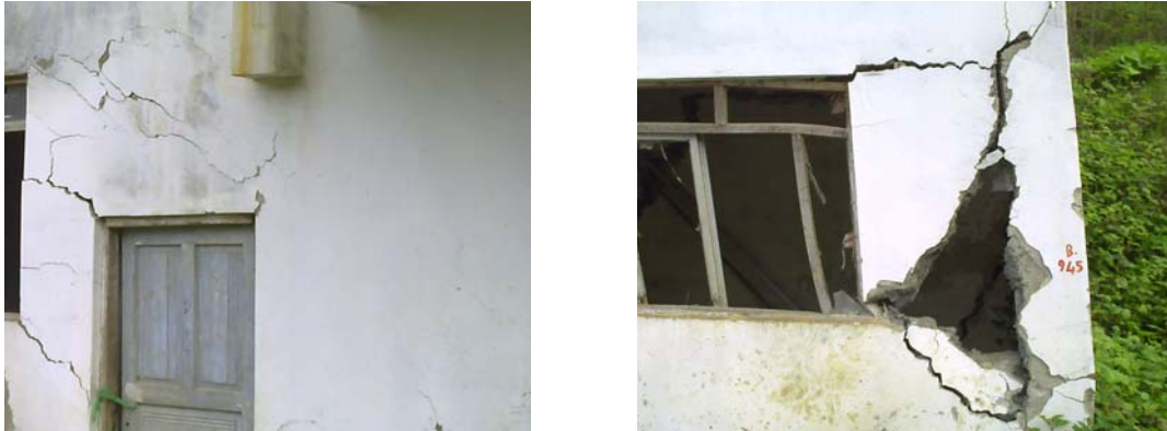
Fig. 1 Detrimental effects of the expansive soil on one storey country house
