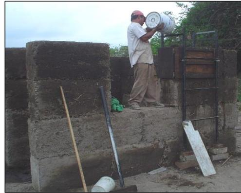
(b) General view of the construction process of the compressed soil blocks and formwork
