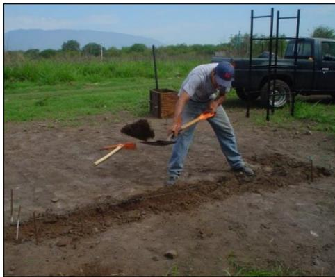
(a) Ditch excavation for the wall's foundation
