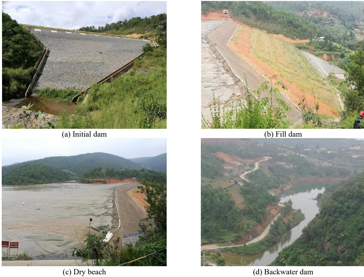
Fig. 1 The components and structures of tailings impoundment
