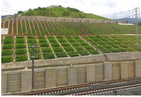
Fig. 1 An anchoring frame structure supporting a multistage slope in Yun-Gui railway, China
