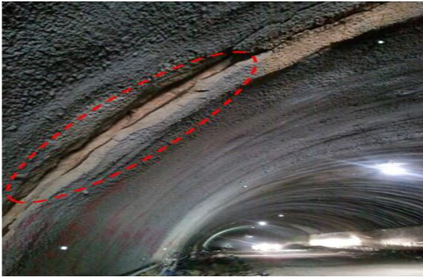
Fig. 16 Convergence of the tunnel under construction
