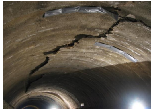
(a) Collapse of tunnel crown
