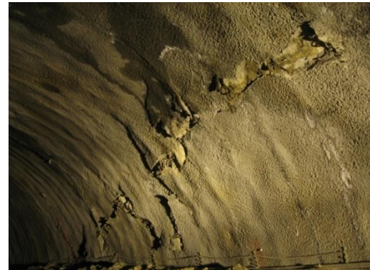
(b) Collapse of tunnel side wall
