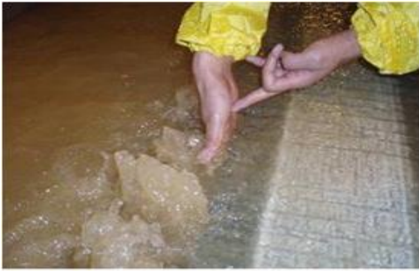
Fig. 13 Upheaval and underwater flow of tunnel pavement
