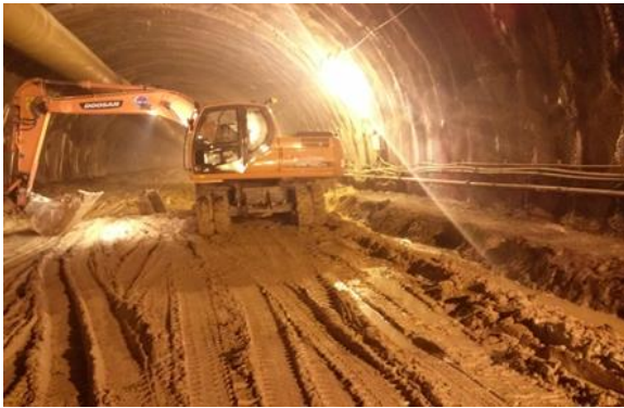
Fig. 14 Geological condition of the tunnel bottom under construction
