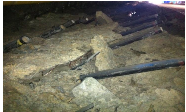
Fig. 11 Upheaval of tunnel bottom under construction
