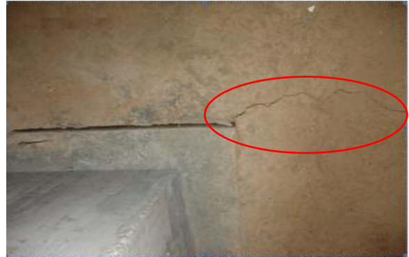
Fig. 8 Loess cracking at the corner of pile cap
