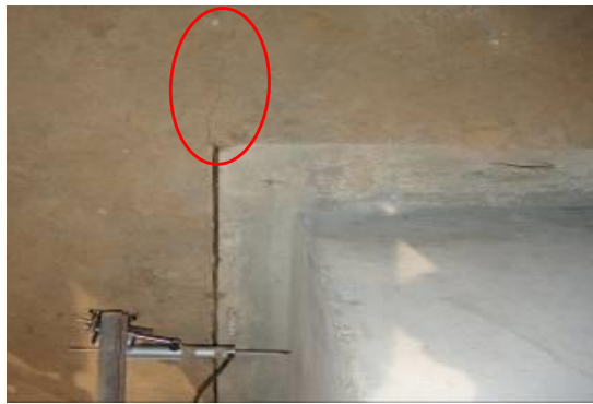
Fig. 8 Loess cracking at the corner of pile cap
