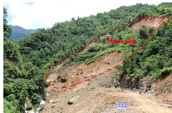
Fig. 1 Instability slip of Daping slope in Fengjie County, Chongqing City, China
