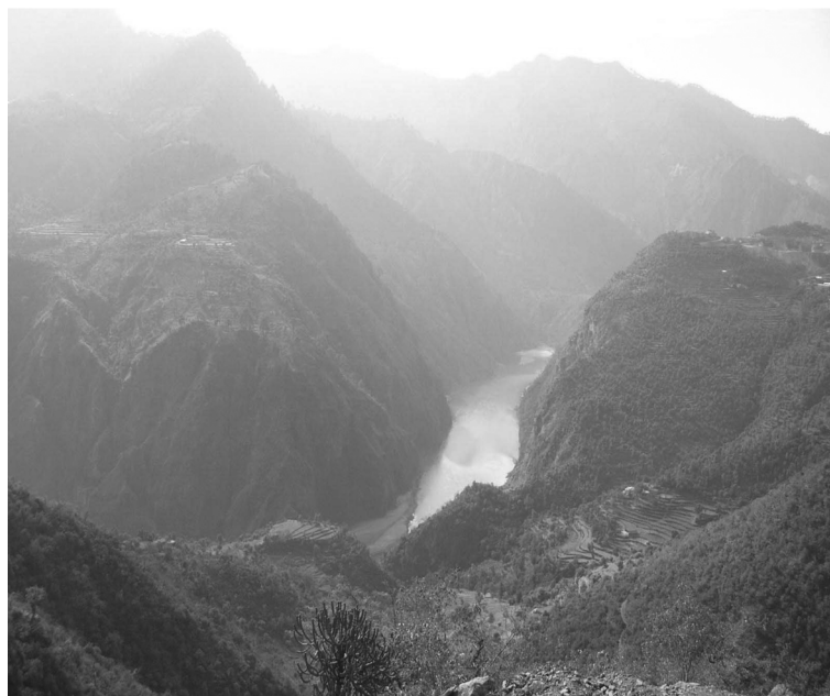
Fig. 2 Photograph showing the proposed bridge site
