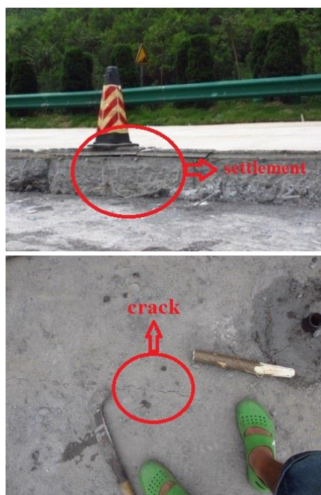
Fig. 10 Uneven settlement and pavement crack of Shao-huai highway
