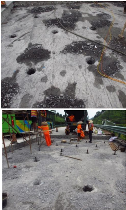
Fig. 16 Site construction drawing of vertical pile grouting
