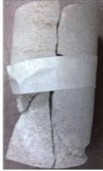
(a) Non prefabricated crack
