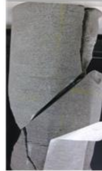
(c) Prefabricated crack of 45° inclination
