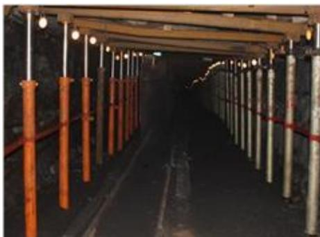
Fig. 13 The effect of “flexible-hard” roadside support
