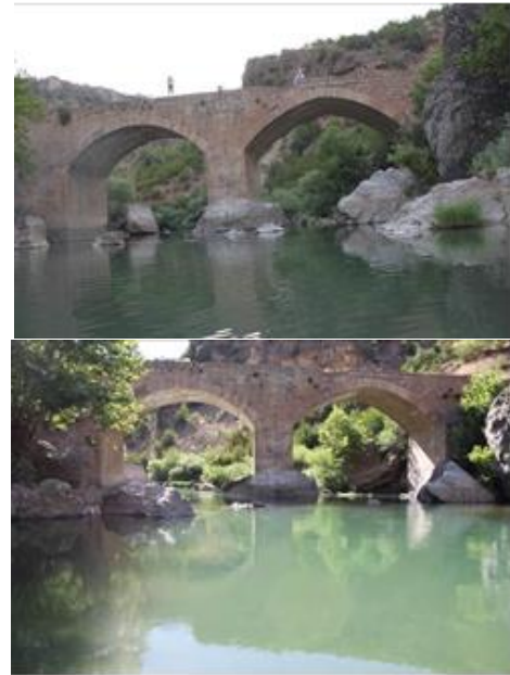
Fig. 1 Göderni two-span historical masonry arch bridge
