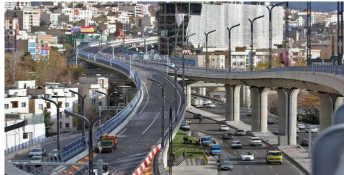
Fig. 2 Sadr Bridge view
