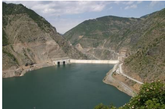
(a) From upstream direction
