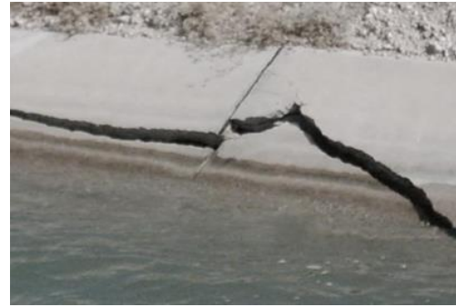
Fig. 1 Failure of Maroon irrigation network canal A concrete lining
