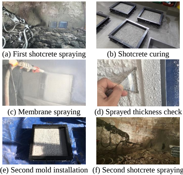
Fig. 13 Preparation of composite shotcrete specimens with sprayed waterproofing membrane
