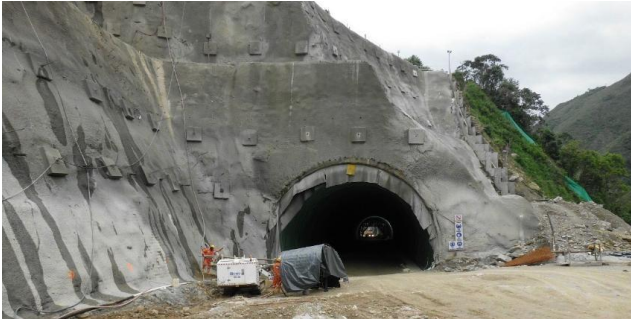
Fig. 11 Low overburden on entrance portal. Tunnel 7, Bogota-Villavicencio road
