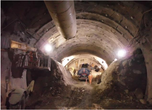
Fig. 3 Tunnelling in terrace soil deposits, tunnel 13 Bogota-Villavicencio road
