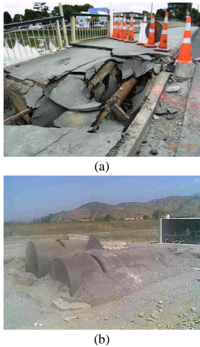
Fig. 1 Damage to industrial components induced by liquefaction, (a) steel buried pipeline (after Yamada et al. 2011) and (b) LPG tanks (after GEER 2010)
