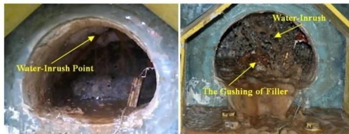
Fig. 11 Inflow of water and mud in Tunnel
