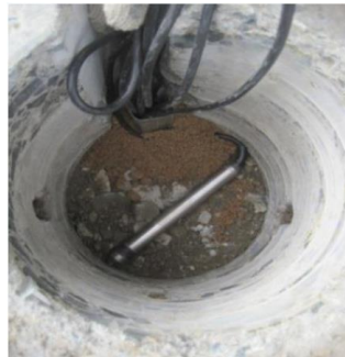
Fig. 5 Installation of sensor into pavement structure
